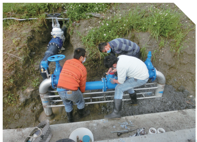
自來水管線施工情形 Water piping work
