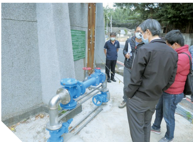
自來水管線設置情形 Installation of water pipes
