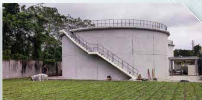
花蓮監獄新建蓄水池 New reservoir built at the Hualien Prison
