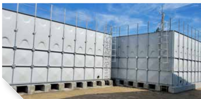
高雄監獄新建蓄水池 New reservoir built at the Kaohsiung Prison
